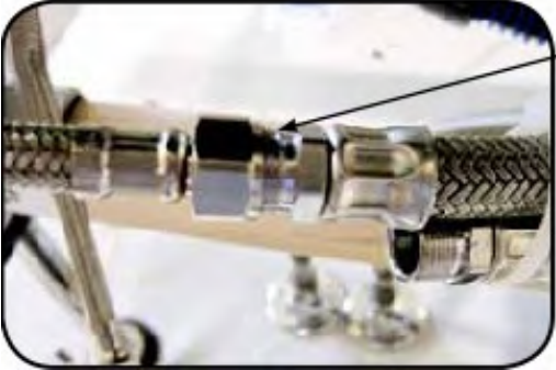
Male/Female fitting connection
